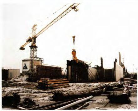
This purification plant in the Rotterdam Botlek area will treat wastewaters of the crop protection chemicals and vinyl chloride monomer plants. In the biological purification stage, powdered activated carbon will be added to the pretreated effluent as an adsorbent. Past experience has shown this addition to be highly effective.
