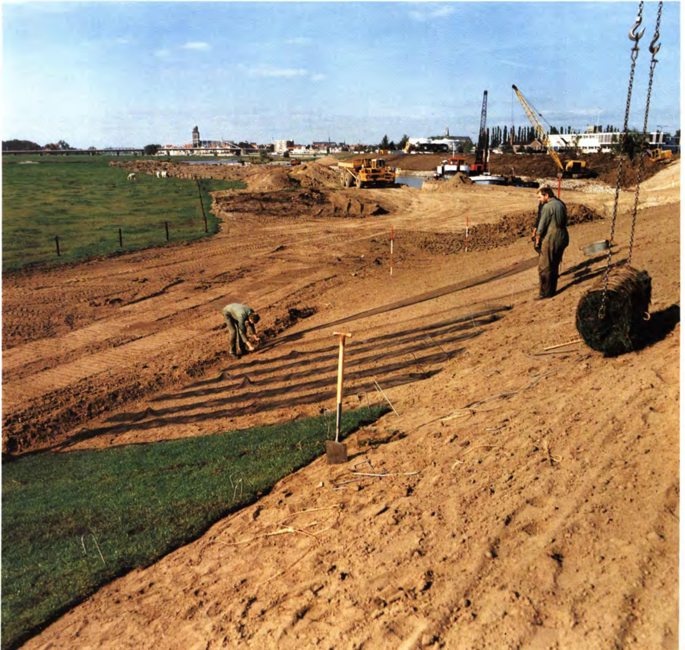
A major application of man-made fibers is as reinforcing materials, which have a wide spectrum of uses. One example is Enkazon®, a reinforced natural turf here providing instant erosion protection on a dike.
