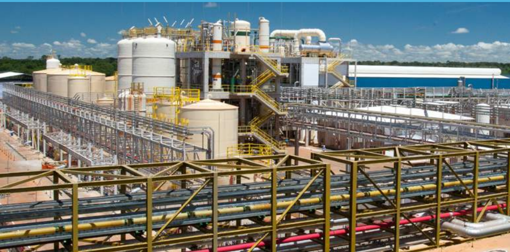
Our Chemical Island sites are integrated with pulp mills and primarily run on renewable excess energy.
